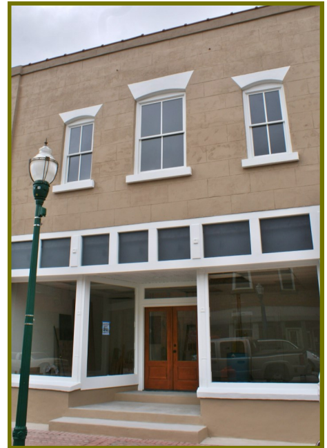
After façade renovations in 2012.
