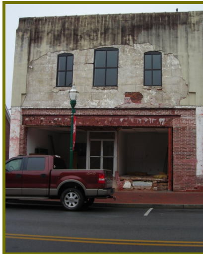
Before façade renovations in 2011.
