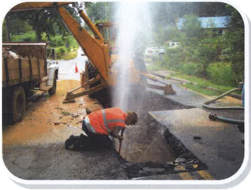
Distribution Crew Repairing a Water Main
