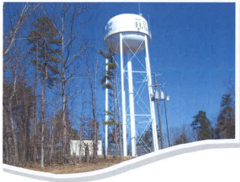
Elevated Storage Tank
