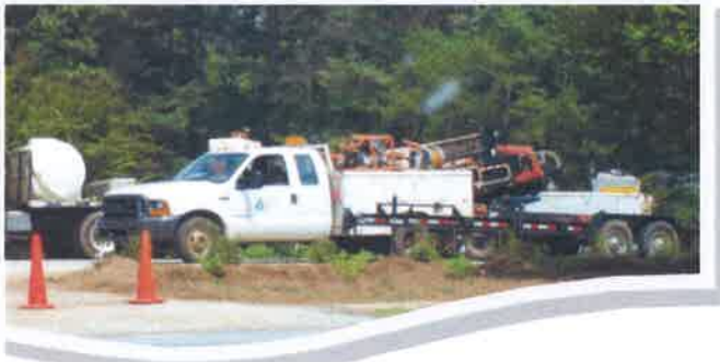
Installing a Gas Distribution Line
