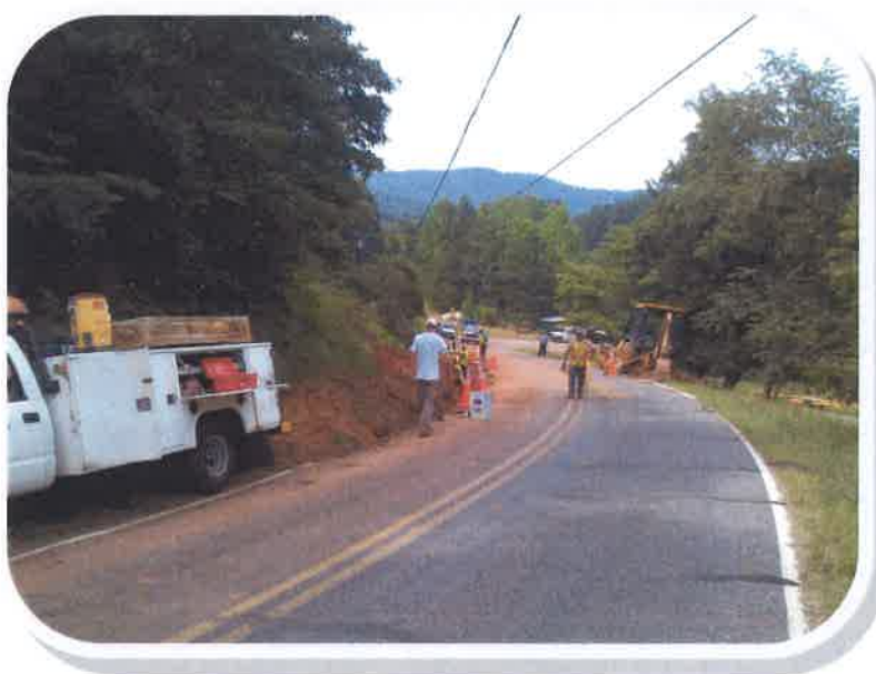
Gas Main Expansion
