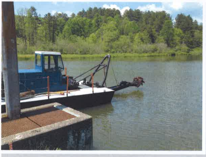
Davidson Creek Reservoir Dam
