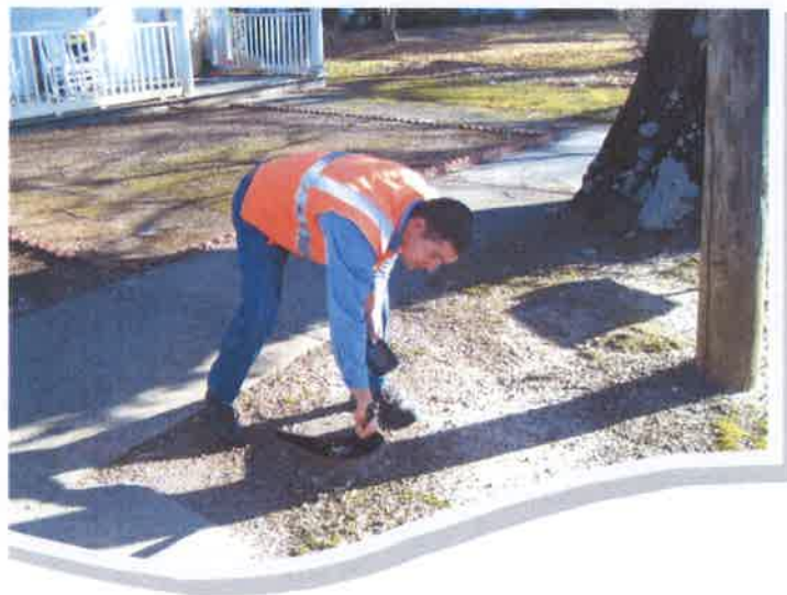
Reading a Water Meter
