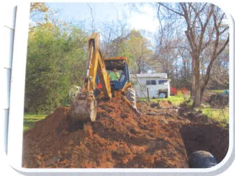
Construction on Storm Water System
