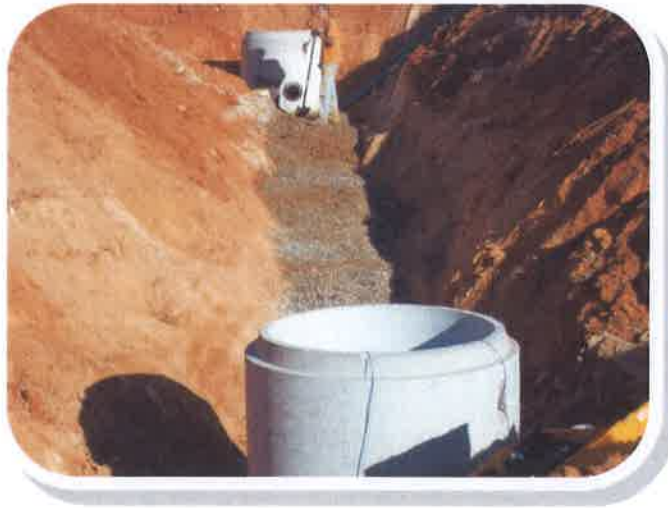
New Construction Inspection
