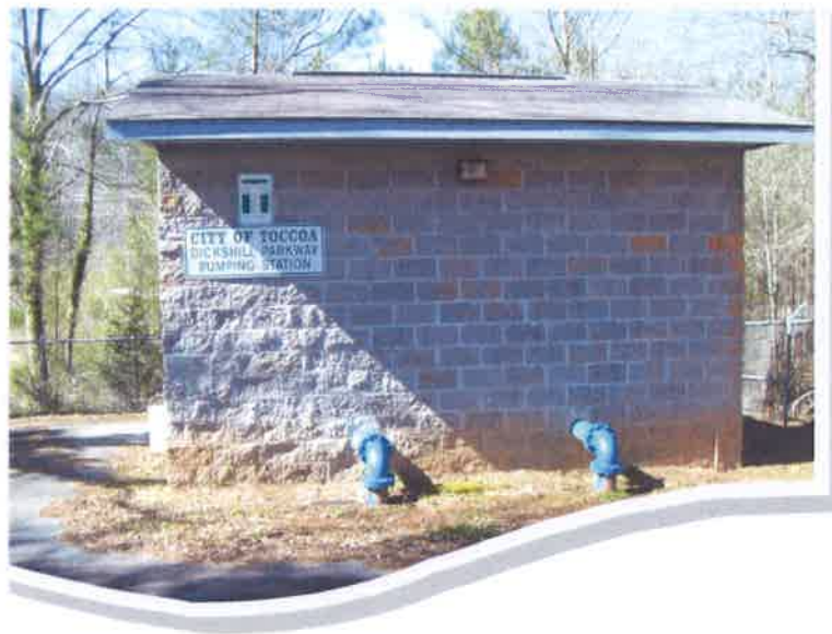
Booster Pump Station
