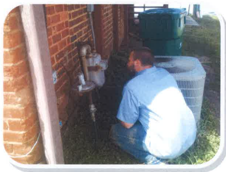
Atmospheric Corrosion Inspection of Gas Meter
