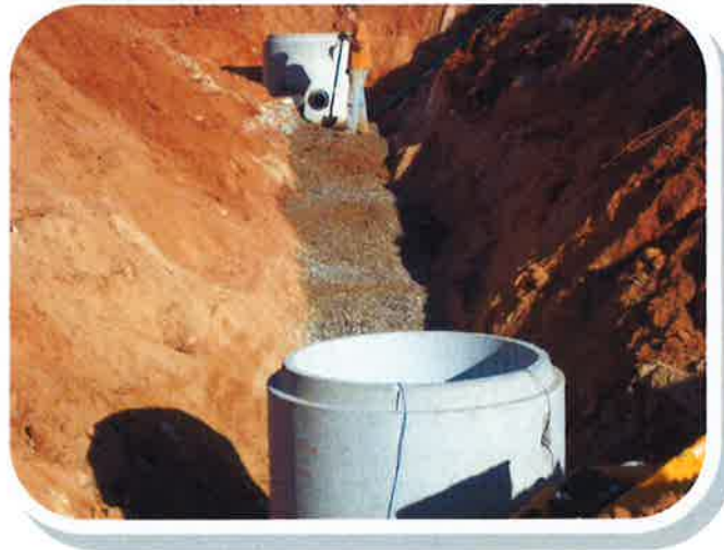
New Construction Inspection
