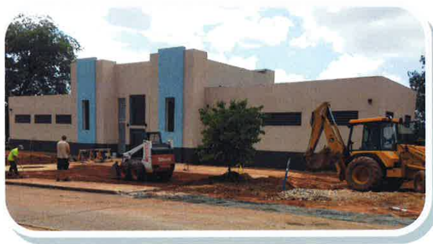
City Pool Bathhouse Construction
