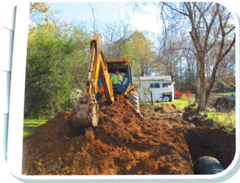
Construction on Storm Water System
