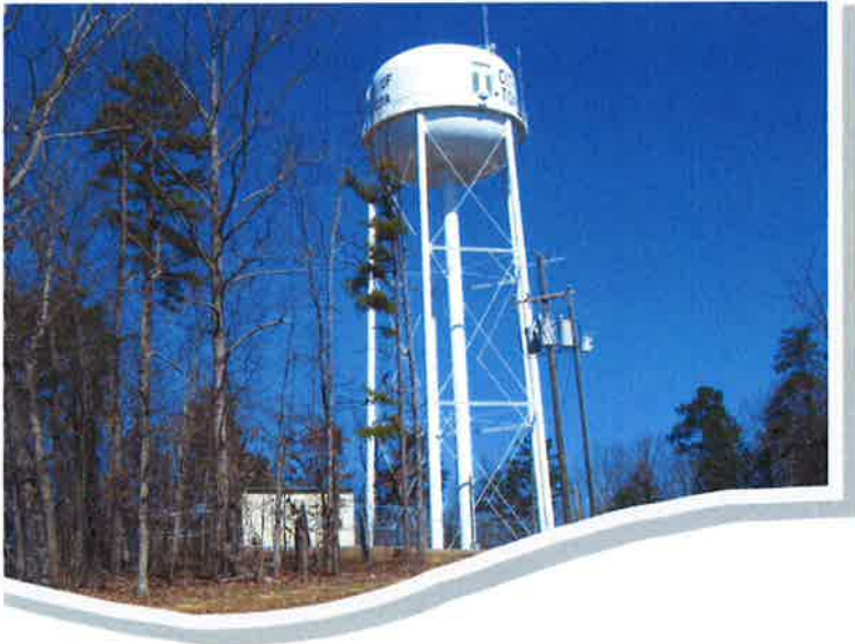
Elevated Storage Tank
