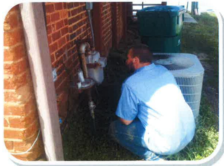
Atmospheric Corrosion Inspection of Gas Meter
