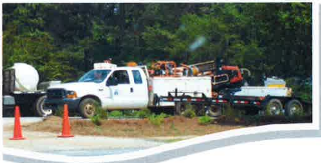
Installing a Gas Distribution Line
