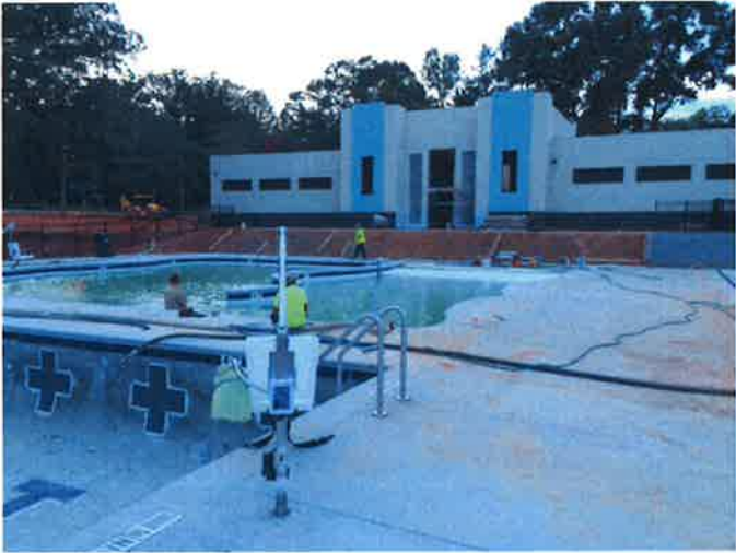
City Pool Construction
