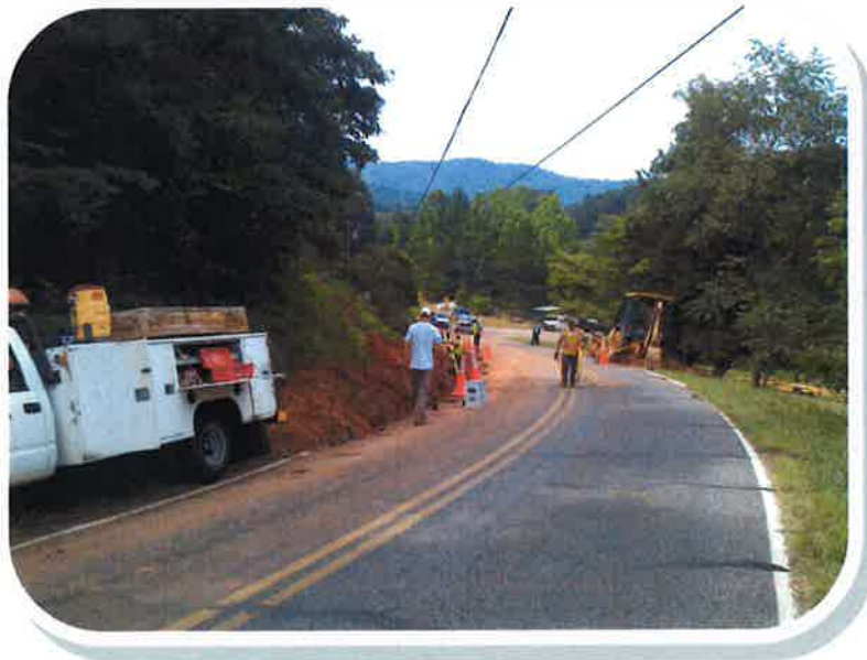
Gas Main Expansion
