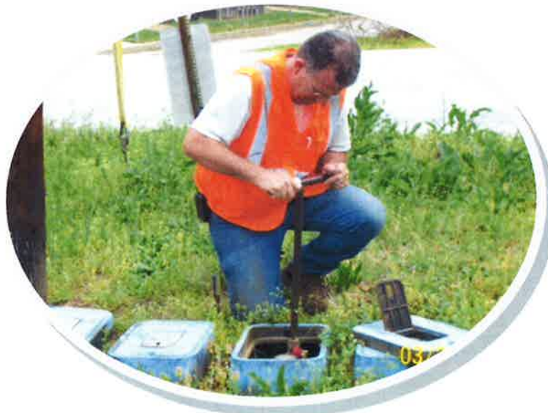
Service Technician Performing Water Leak Check
