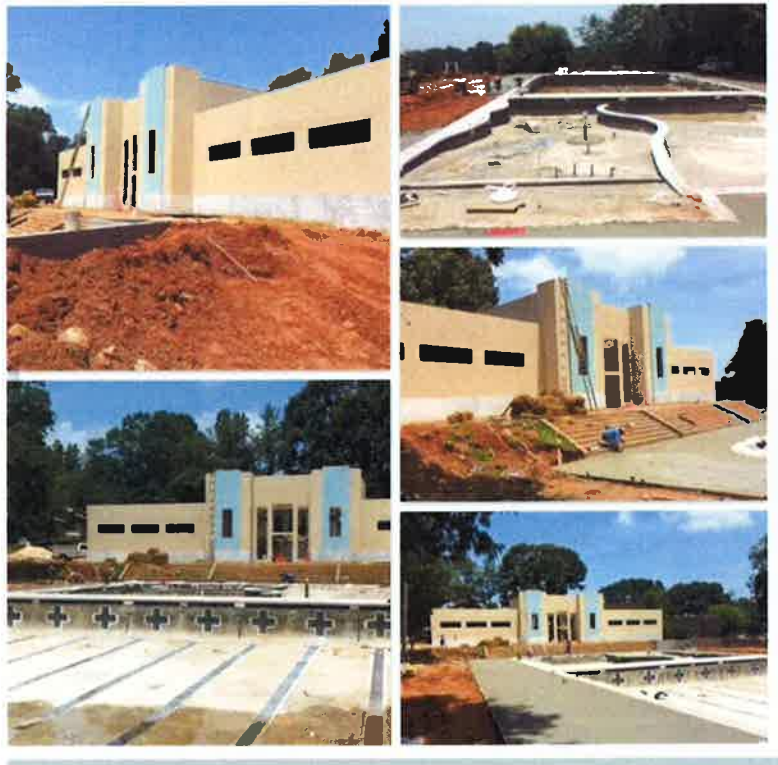
Construction of the City Pool
