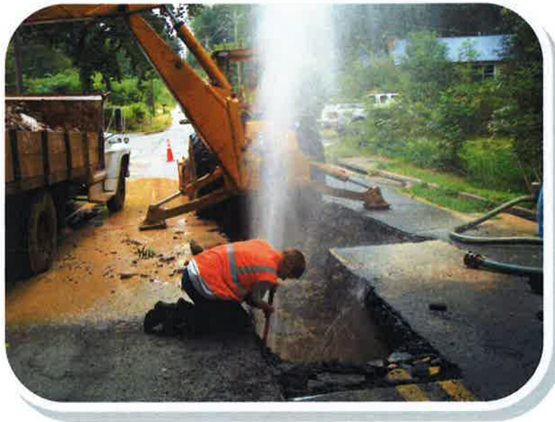
Distribution Crew Repairing a Water Main
