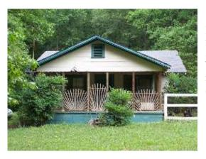
Porch with inappropriate addition of balustrade in an incompatible style.
