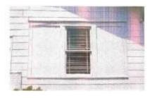
Example of inappropriately sized window infill that is not characteristic of the building.
